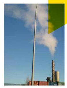
The drying of the aggregates generates steam which can be seen being emitted from the stack of the plant. This may sometimes appear dark if the sun is sitting behind the stack.
